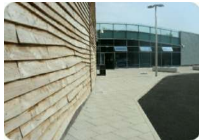
Colwyn Bay, Saron paving and kerb
