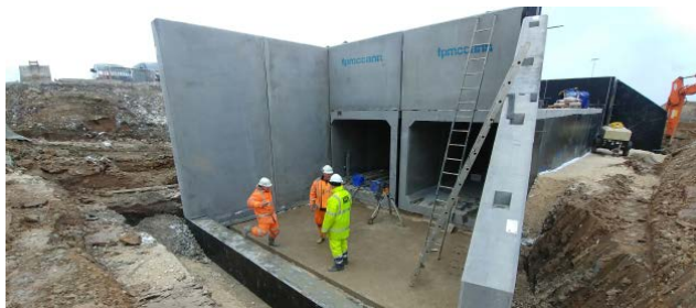
Box culvert with wing walls
