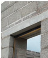
Concrete lintel as used traditionally in construction.
